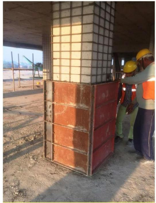
**FIGURE 6: PROVIDING SHUTTERING AROUND THE COLUMN.**
