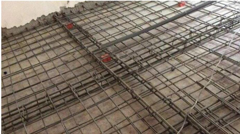
**FIGURE 8: REINFORCEMENT MESH BOTTOM (OR TOP) OF THE FLOOR SLAB, THE MAIN REINFORCEMENT IS ANCHORED INTO THE BEAM WITH CHEMICAL ANCHORING.**
